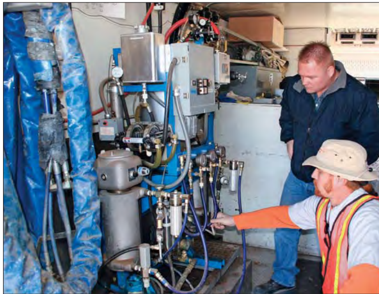
Don McDowell looks on as operations manager Tom Van Duinen checks the pumping system. This is where the epoxy components get their final heating and pressurization.
